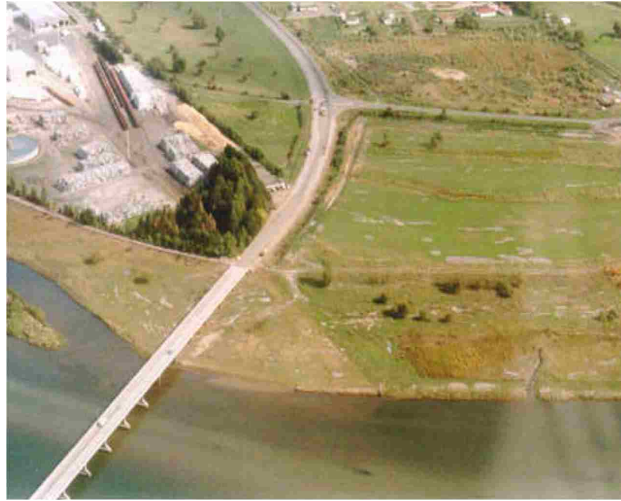
Figure 1.2: Northern approach to Landing Road Bridge two days after the Edgecumbe event. Ejected sand is visible on the ground surface (Berrill and Yasuda, 2002).
