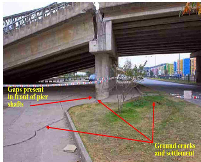
Figure 6.3: Portion of northeast approach to Puente Llacolén affected by liquefaction-induced ground deformation (FHWA, 2011).
