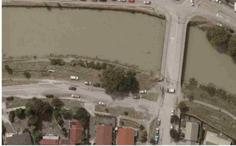
Figure 1.7: Avondale Road Bridge after the Christchurch event. Lateral spreading cracks are visible near the southern approach and along the river bank (LINZ, 2011).
